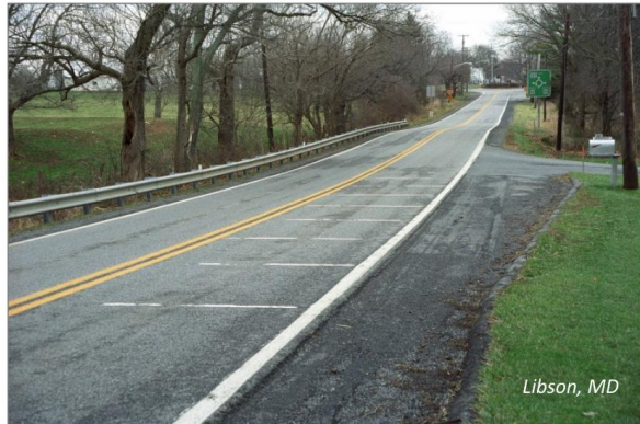
Exhibit 2 – Example of a Traverse Rumble Strip
