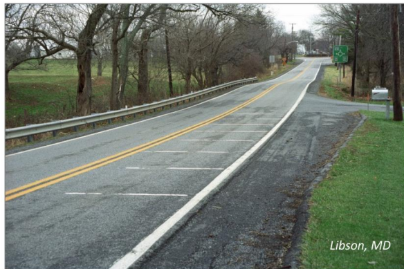
Exhibit 2 – Example of a Traverse Rumble Strip
