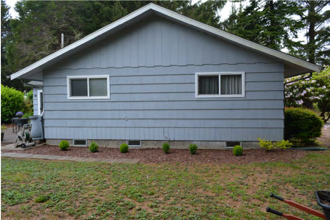
View: Side / east facade, view to the west
