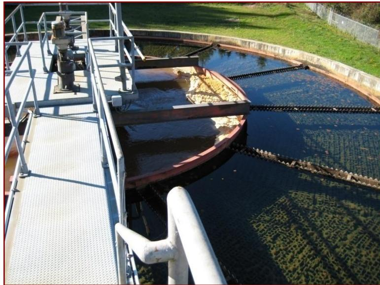
A second clariflocculator was added in 1978-79 as part of an upgrade to the plant and to increase the overall capacity of the water treatment facility. The second unit is of similar size and construction to the first. However, the newer clariflocculator has settled over the years and does not operate properly as the water service in the tank is no longer level with the overflow launders around the tank.
