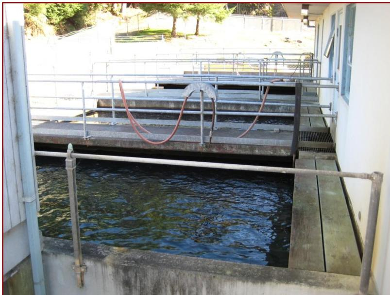
Filter No. 4 has historically had problems related to structural or foundation issues. These issues have manifested themselves in cracks in the concrete that propagate into the clay underdrains. The filter has consistently experienced short circuiting and turbidity break through as a result of the damaged under-drain system. Replacement underdrain tiles that match the existing tiles are not readily available today.
