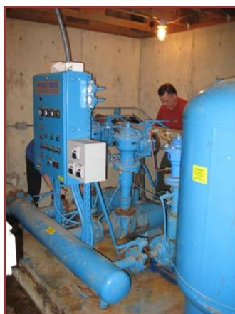
Suction pressures range from 40 to 47 psi depending on pumping rate and water level in the Main Storage Tanks. Discharge pressure of 80 psi in the pressure tank (HGL = 350') provides a pressure of about 52 psi at the top of the service area (elev. 230' ±). The service area is relatively small and is unlikely to increase in size unless service outside the UGB is provided in the future.
