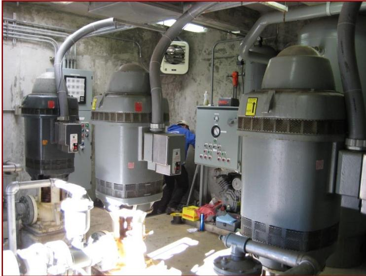
There are three pumps located within the Siletz intake. Each pump has a 200 horsepower, 460-volt, 3-phase, 1800-rpm vertical motor manufactured by U.S. Motors. Each pump is a Fairbanks Morse 12M, 7-stage, CT head vertical turbine pump rated for 1000 gpm at 560 feet total dynamic head (TDH). With two pumps running at once the station output is approximately 2200 gpm with a discharge pressure exceeding 200 psi.
