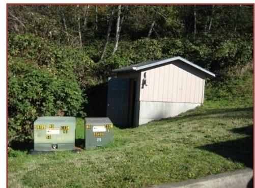
The Lakewood BPS contains pumps which likely are at the end of their expected service life and which are too small to provide fire protection in the service area. The Lakewood BPS should be replaced as soon as possible during the planning period with equipment designed to provide normal service to 50 lots and to provide fire flows. Discharge pressure should be reduced.
