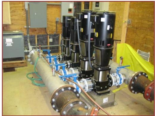
The station equipment is a Grundfos Booster PAQ with on/off control based on pressure in a hydro-pneumatic tank located inside the building. Power supply is 460 volt, 3 phase. Four Grundfos vertical multi-stage centrifugal pumps are utilized including two 25Hp CR90-2-2 rated for 440 gpm at 155' TDH, and two 7.5Hp CRE 16-40 rated for 75 gpm at 230' TDH at full speed. Variable speed drives are used to provide lower flows for typical daily demands.
