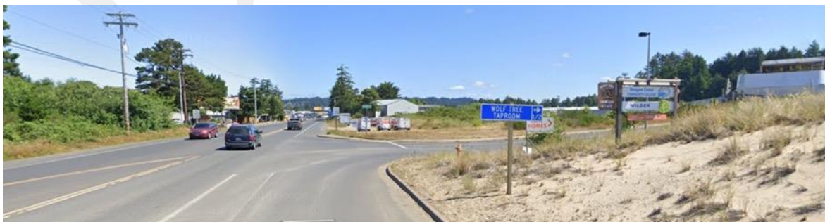
US 101 northbound approaching the intersection of SE 40th St., access to Wilder and the OCCC
