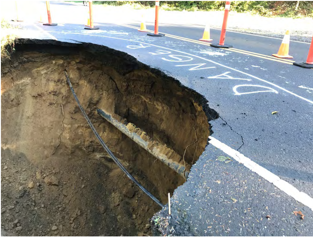
Photo 8. Exposed utilities and headscarp looking northeast.
