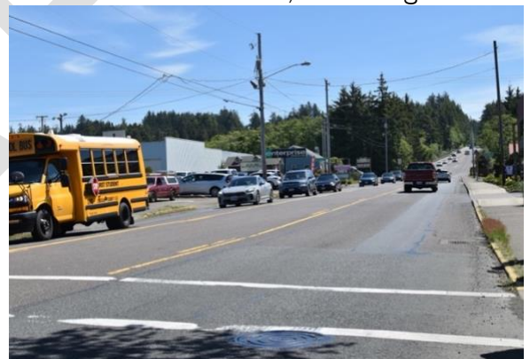
Narrow sidewalks along US 20. Crosswalk at NE Eads Street and US 20 crossing three lanes.
