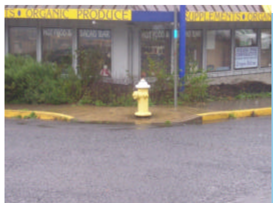
Sidewalk fire hydrant on ramp, preventing full use of the curb ramp on SW 2nd Street
