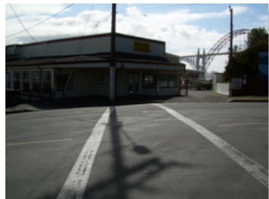
Some crosswalks are difficult to see due to minimal markings
