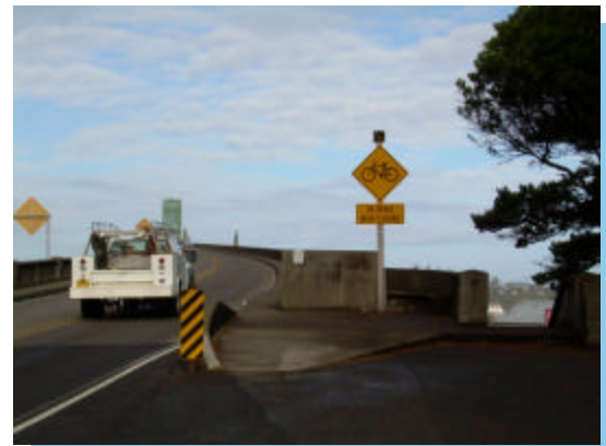
Existing signage for crossing Yaquina Bay Bridge
