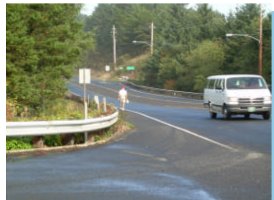
Debris in the bikeway on U.S. 101
