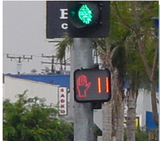
Pedestrian crossing countdown signal
