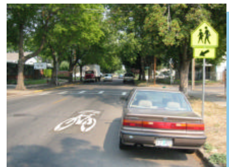
Sharrow placement on a local street
