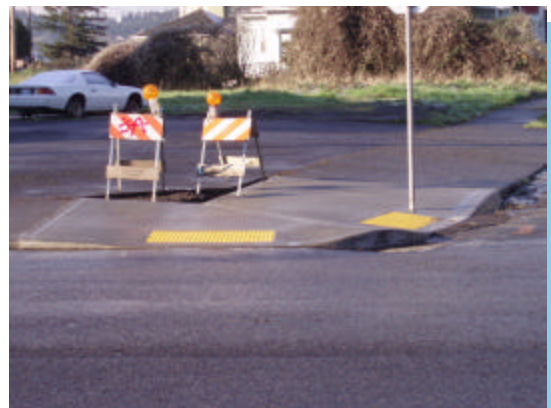
Dual curb ramps with detectable warning strips
