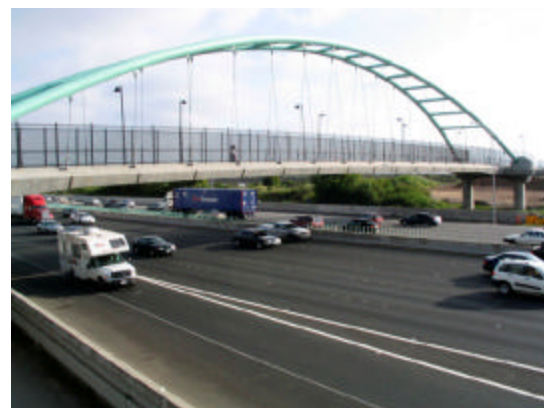
Type 4 Grade-Separated Overcrossing
