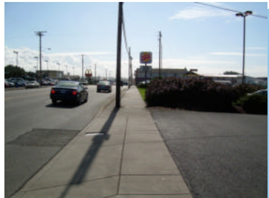
Sidewalk on U.S. 101 near 15th Street
