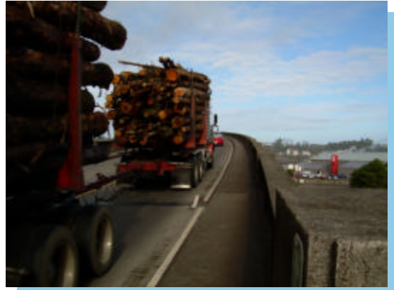
Yaquina Bay Bridge sidewalk with truck traffic
