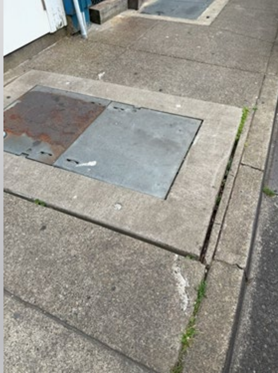
Example Concrete Vault Trip Hazards
