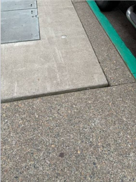
Example Concrete Vault Trip Hazards
