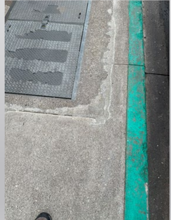
Properly Ground Concrete to Match Sidewalk Grade
