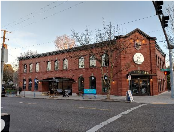
New-construction corner businesses: stores and offices above
