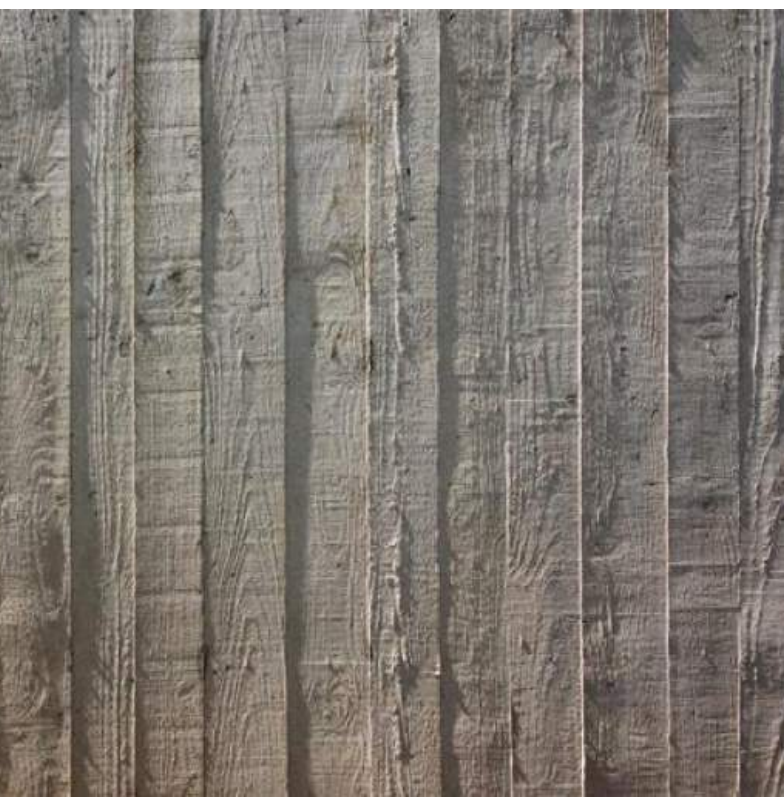
C-1 - BOARD FORMED SITE WALL - COLOR: STONE
