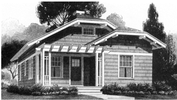
Multiple distinct low pitched gabled roofs (with clipped gables/jerkinhead roof)
