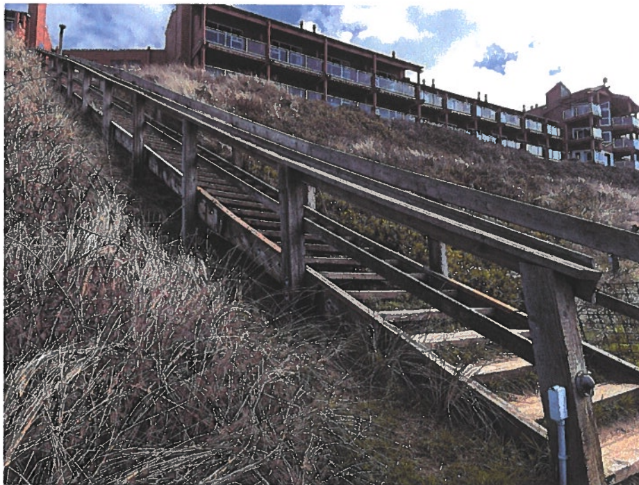
Photo 4: Access Site 4 – Access Structure on Steep Slope
