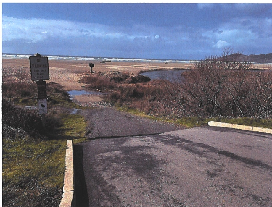
Photo 8: Access Site 8 – Ramp and Creek Crossing
