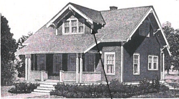
Side gabled roof with front gabled roof dormer
