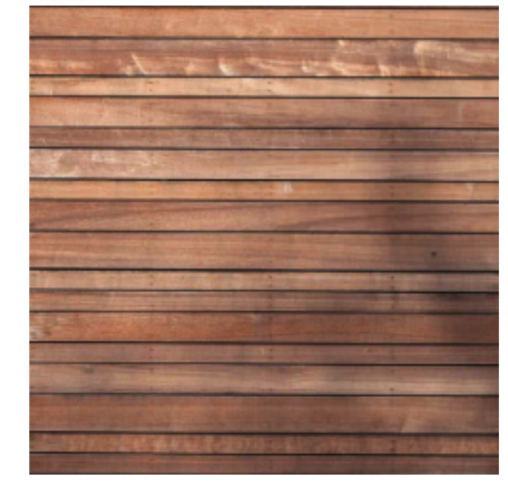
S-2 - PLANK SIDING - CLEAR STAIN
