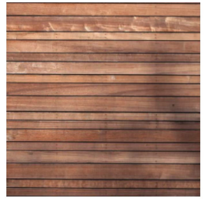
S-2 - PLANK SIDING - CLEAR STAIN
