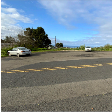
114. Pullout on Lighthouse Drive (city-owned section), 10-12 spots delineated in faded paint. Pavement deteriorated with patches. - Looking South
