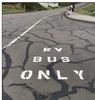
BLM uses crack sealing techniques to repair cracks in the pavement at the ONA.
