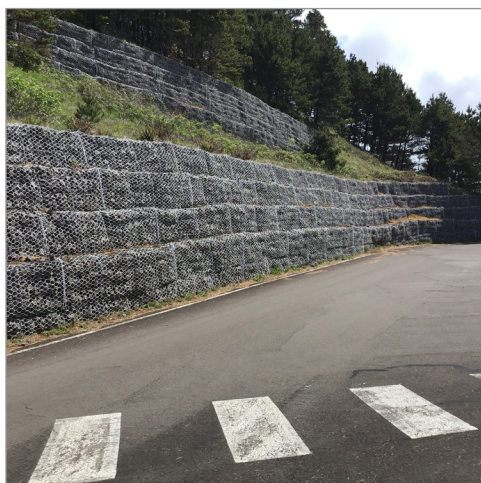
36. Erosion control retaining wall "cages" at Quarry Cove - Looking East
