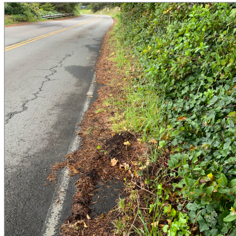
119. Pavement width on north side of Lighthouse Drive (city-owned section), overgrown shoulder estimated 3ft width - Looking West
