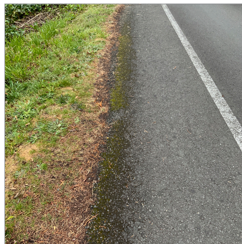
120. Pavement width on south side of Lighthouse Drive (city-owned section), 39" fog line to pavement edge - Looking West
