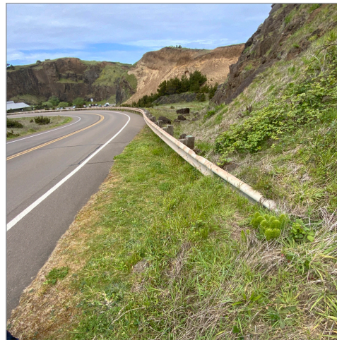
143. Guardrail buried in vegetation (typical of most guardrail ends) - Looking West
