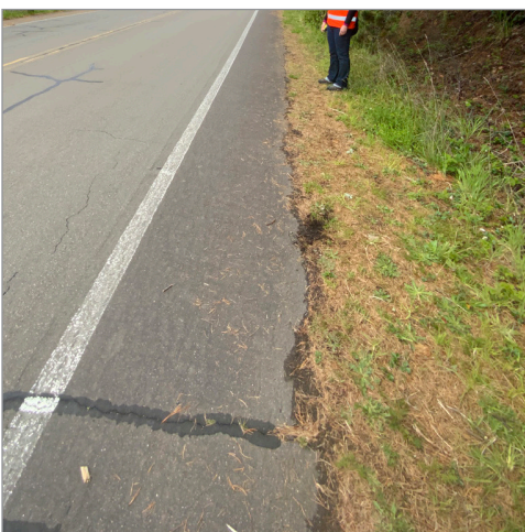
140. Lighthouse Drive approaching S-curves, 3' shoulder fog line to edge of visible pavement on north side, 4.5' shoulder fog line to edge of pavement on south side - Looking West
