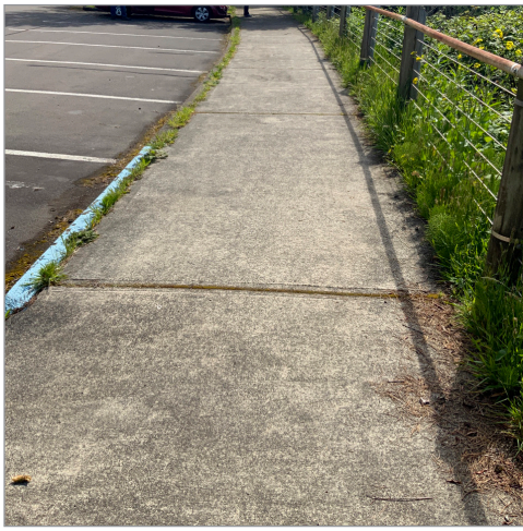
129. ADA stalls in Quarry Cove overflow parking lot, 31 regular stalls plus 2 ADA stalls. Sidewalk entire length of lot, 58" wide - Looking South
