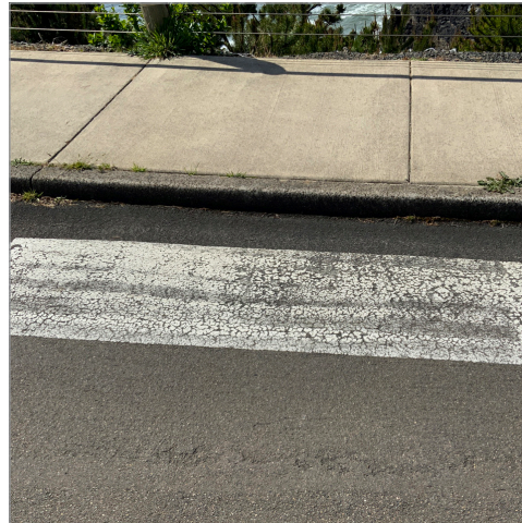
134. Crosswalk across upper parking lot at Quarry Cove, no curb ramps - Looking South
