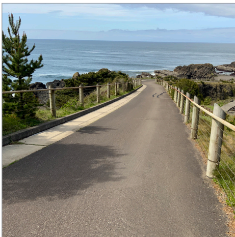
131. Quarry Cove ADA access road, 12' pavement, 32" sidewalk, - Looking Southwest
