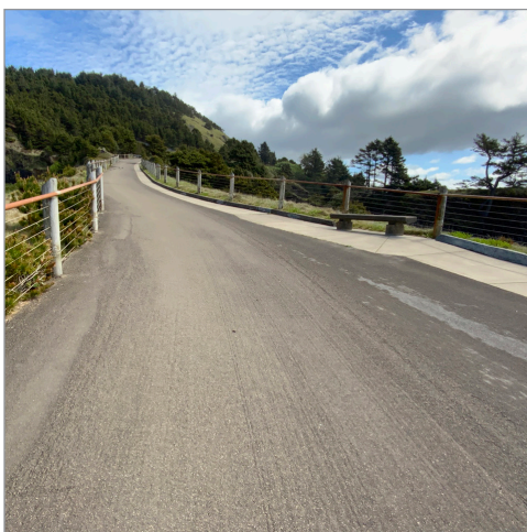
132. Quarry Cove ADA access road, 21' pavement, 6' sidewalk, - Looking Northeast
