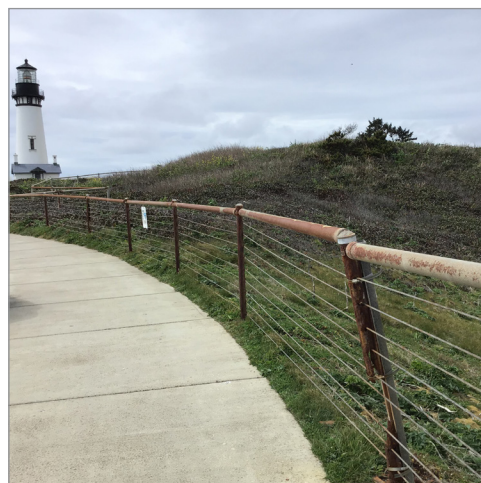
96. Sidewalk around Lighthouse Circle. Railing rusted/deteriorating - Looking West
