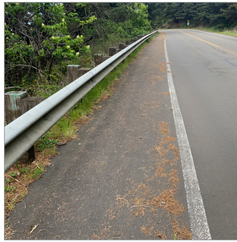
141. Lighthouse Drive approaching S-curves, 3' shoulder fog line to edge of visible pavement on north side, 4.5' shoulder fog line to edge of pavement on south side - Looking West
