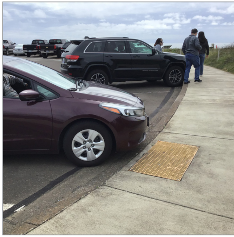
97. ADA curb ramp blocked by a parked vehicle in Lighthouse Circle parking lot - Looking West
