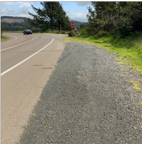
139. Pullout/enlarged shoulder (not signed) on south side of Lighthouse Drive west of Quarry Cove intersection, 15' width edge of pavement to edge of mowing - Looking East
