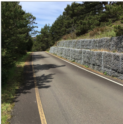
43. Additional retaining wall cages along entrance road to Quarry Cove - Looking West
