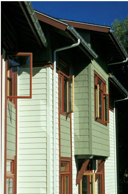
LEED Silver Residence Hall at Lewis & Clark College
