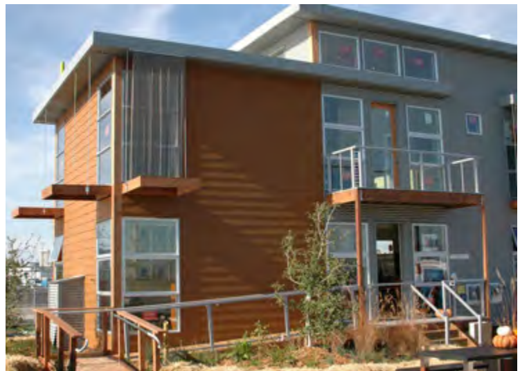
The NowHouse uses SIPs technology for the entire construction.
