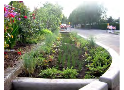
Photo top: deep bioswale between a parking lot and the roadway; Photo bottom: a bioswale integrated with traffic calming
