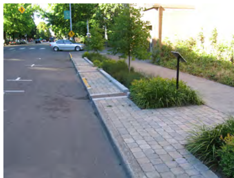
The bioswale above is set back from the roadway to accommodate people getting into and out of their vehicles.
