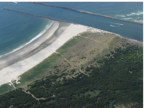
Changes in shoreline positions adjacent to jetties
