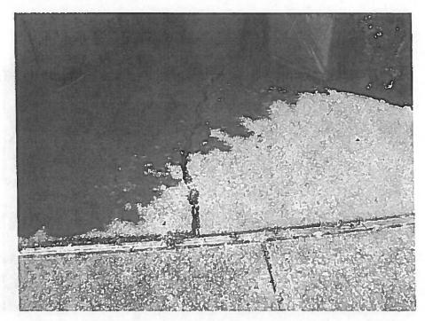
Photo 4 - Slight settlement of concrete driveway slab and a break in the concrete likely due to a soft subgrade.
