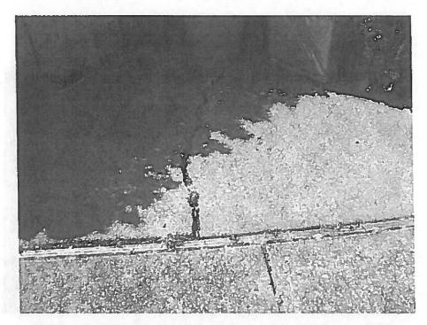
Photo 4 - Slight settlement of concrete driveway slab and a break in the concrete likely due to a soft subgrade.
