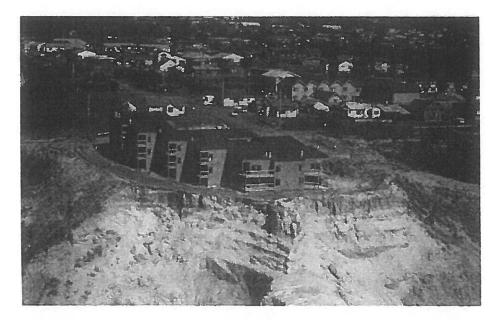
**Figure 9.8** This site on a rapidly eroding bluff with landslides on both sides was extremely precarious for development. The southwestern portion of the structure (lower right) is already beginning to tilt.
