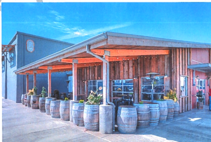
Recent brewpub development in Tillamook's Hoquarton overlay zone incorporating industrial aesthetic
