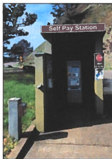
Utilities are provided near the entrance station for the AFM.
