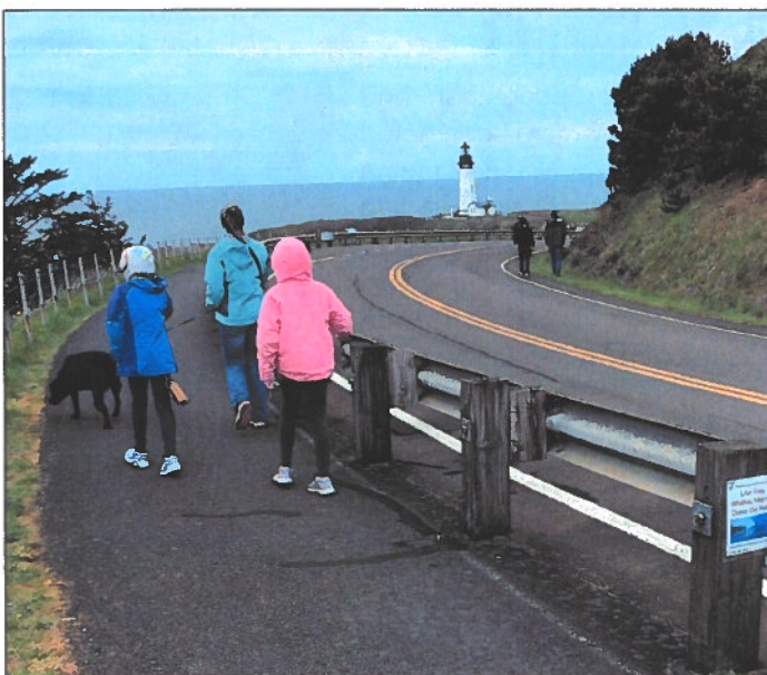
A continuous, protected pedestrian facility along the length of Lighthouse Drive is desired to improve pedestrian safety. Enhanced wayfinding may be needed to direct pedestrians to the path and reduce the potential for pedestrians in the roadway.
