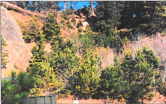
In the past, landslides have occurred on this hillside near the entrance station, blocking traffic and staff exit from the fee booth.
