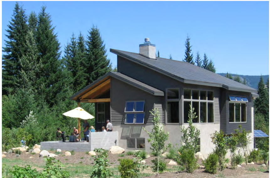
The LEED-H Silver Home at Parkdale, Oregon, Built by Neil Kelly homes
