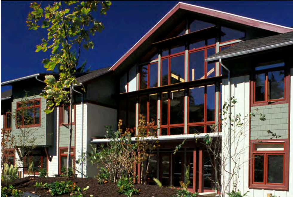
Student Apartments, Lewis & Clark University, Portland, OR - use of bays, trims, and massing to break down the scale of multi-family structures
