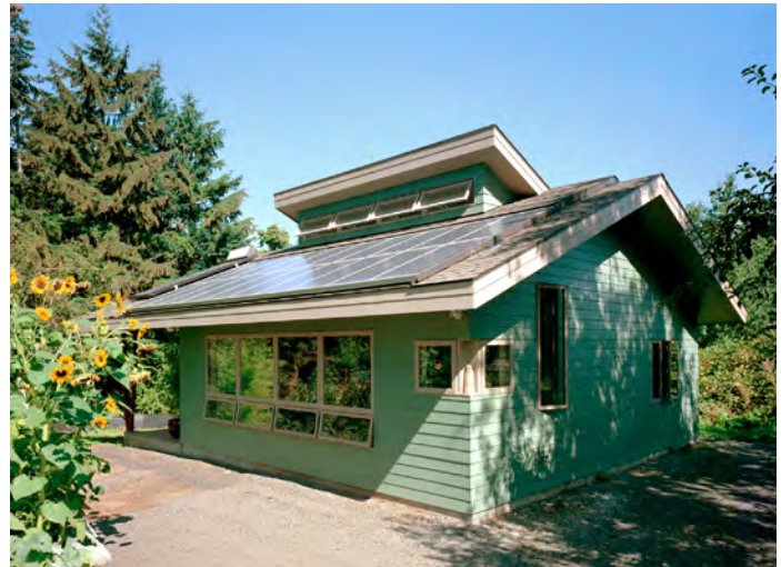
The Rose house was built with SIPs for the roof. (Portland, OR)
