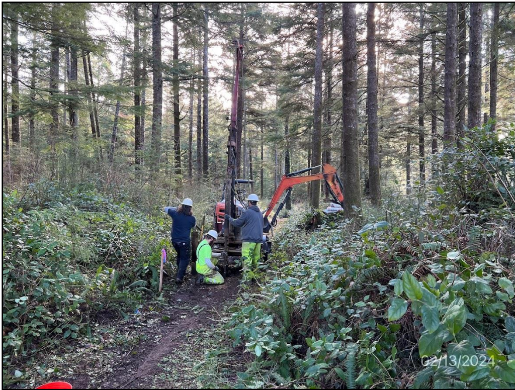
Photo 2: Drill rig setup at exploration location B-10, looking southwest.
