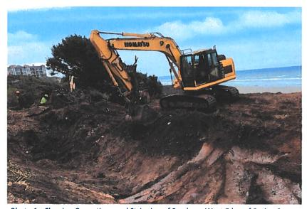
Photo 1 - Clearing Operations and Stripping of Swale on West Edge of Spring Street
