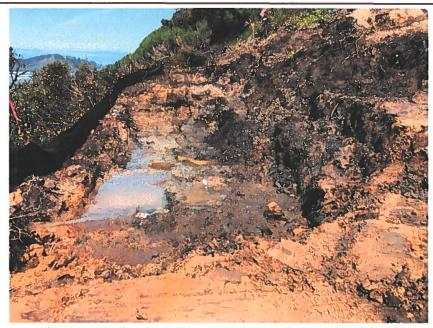
Photo 3 - View of MSE Foundation Excavation. Bedrock Exposure at Right
