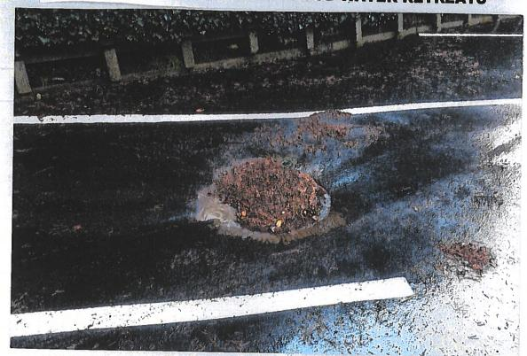
LEAKING WATER FROM DRAIN LINE FAULT ON TO LOWER DRIVE
