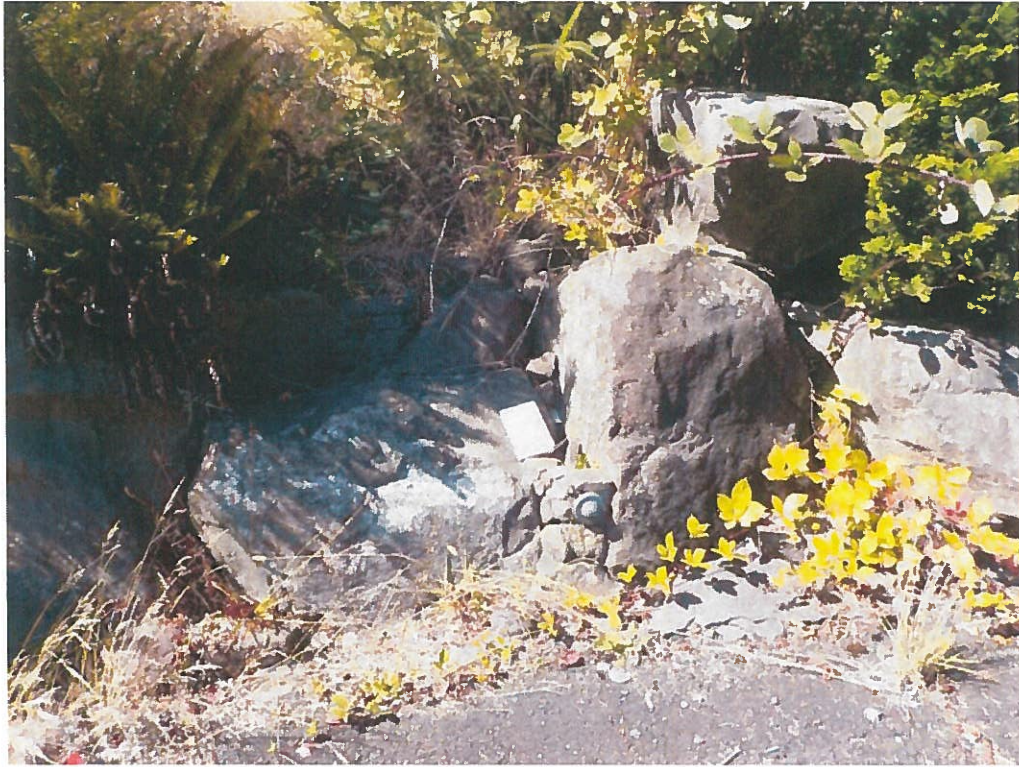
Photo 13 – View of the stacked boulder wall along the eastern driveway.
