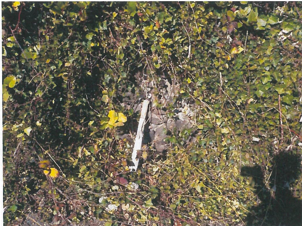
Photo 12 – Close up view of the wet stacked rockery wall at the base of the steep slope along the northern portion of the site.
