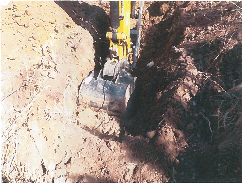
Photo 6 – View of buried wires exposed during the excavation of Test Pit 2.
