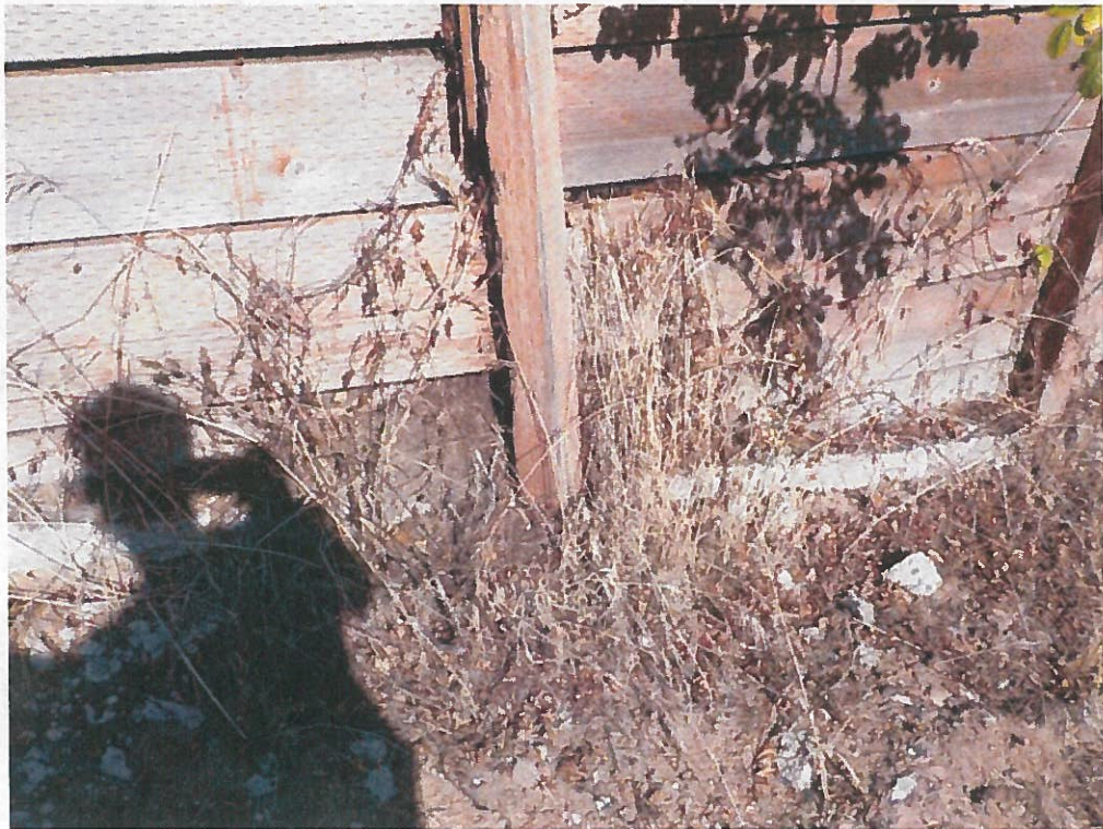
Photo 14 – Close up view of damage typical of the wood lagging wall.
