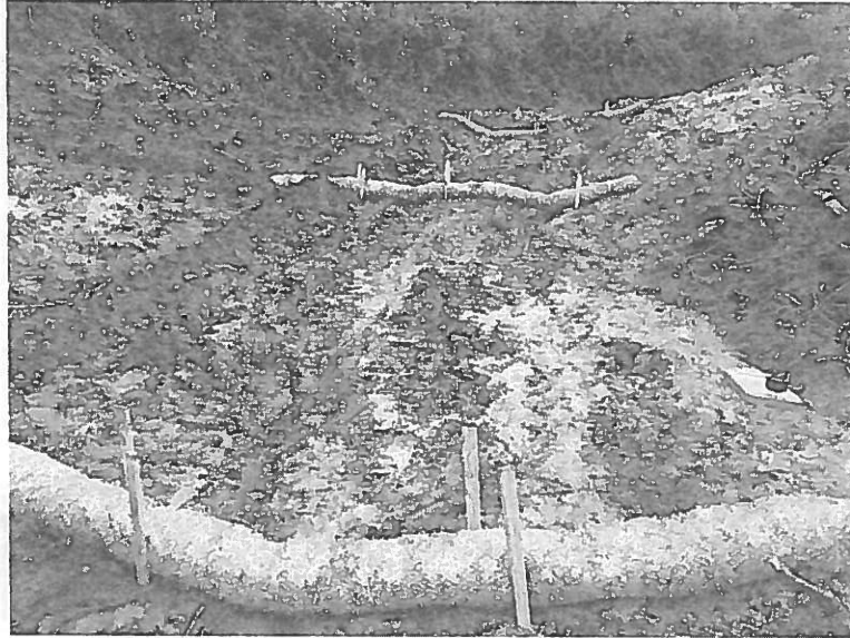
Figure 2. Wattle Construction - slope must be regraded smooth with 2 to 4-percent gradient downslope.
