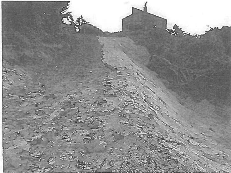
Figure 1. Erosion control blanket used in construction (orange lines indicate seam locations).
