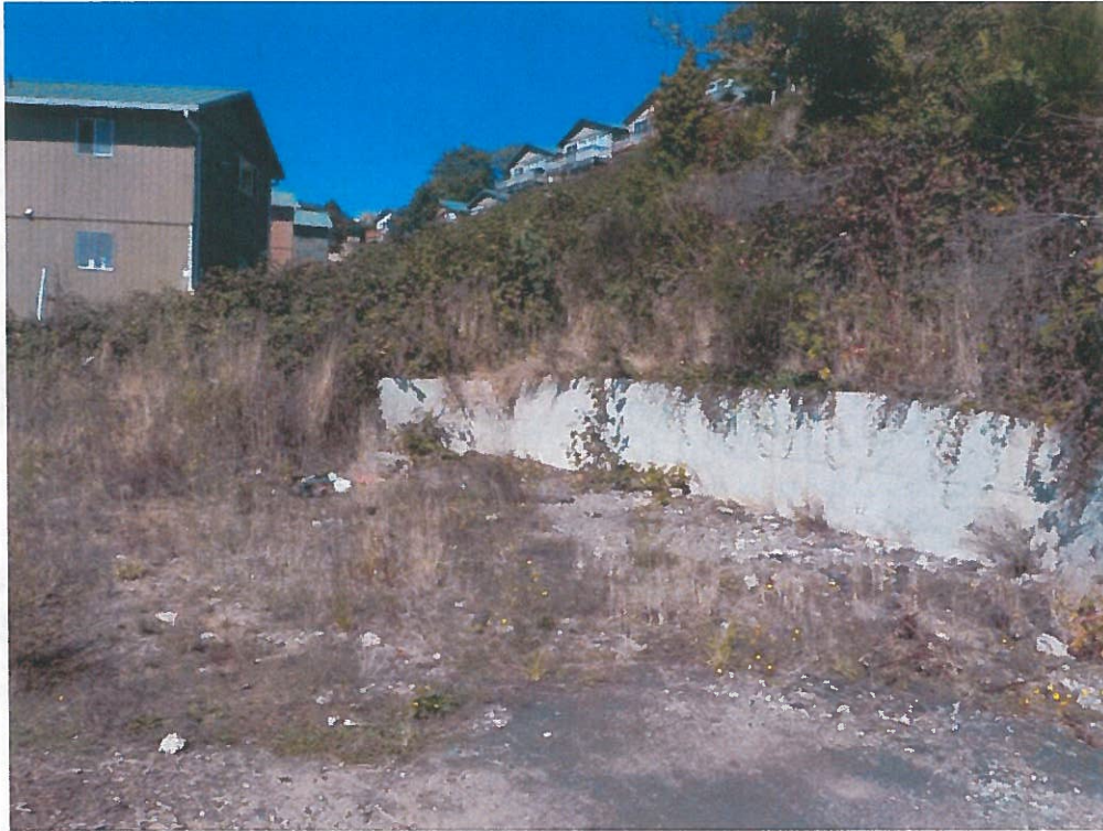
Photo 11 – View of the concrete wall near the northwest corner of the site.
