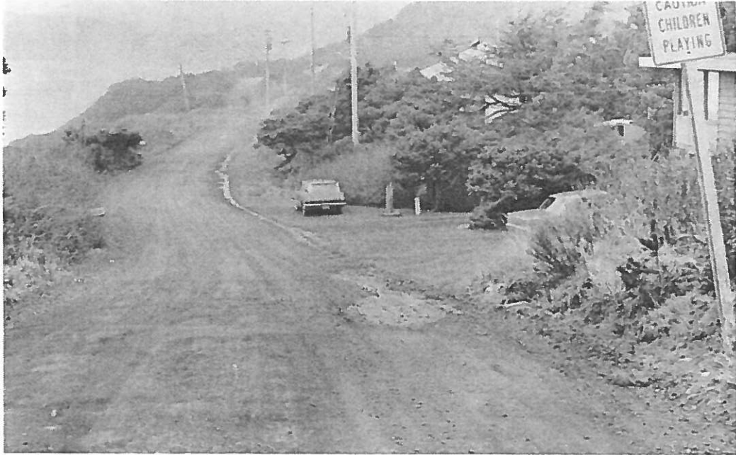
Photo 45. Spring Street dislocated by landslide movement. Water flowing down right side of street comes from spring, indicating the disturbed subsurface drainage of the landslide mass.
