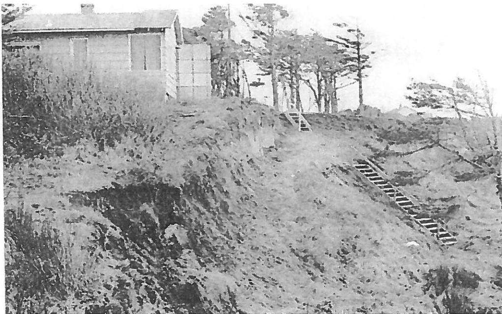
Photo 44. Close-up of part of the large landslide scarp exposed behind house on Spring Street. Extensive damage to house began in 1961 and slide mass continues to be unstable.
