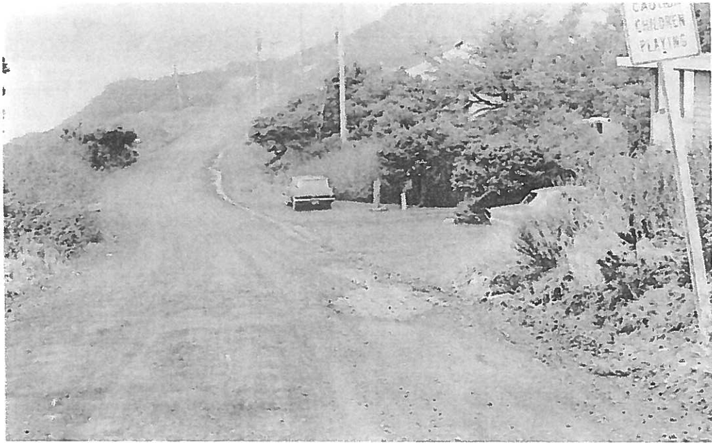
Photo 45. Spring Street dislocated by landslide movement. Water flowing down right side of street comes from spring, indicating the disturbed subsurface drainage of the landslide mass.
