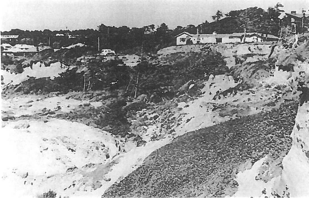
Photo 43. Active landslide at Spring Street just north of Jumpoff Joe in Newport creates a jumble of unstable ground involving many acres of land.
