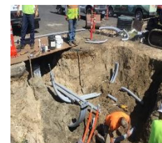
Ferry Slip Road Utility Line Undergrounding
