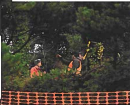
Heavy brush and trees removed from the east side of the skatepark in 2018.
