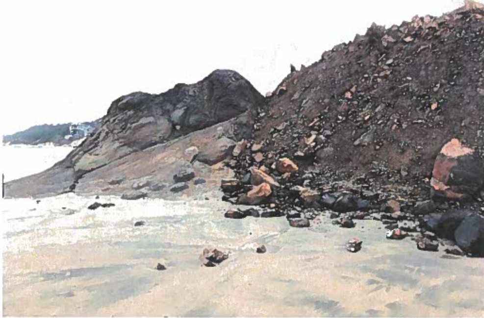
Photo 11. Slide debris pushed up against a rock outcrop at the toe in the central portion of the slide looking northeast.
