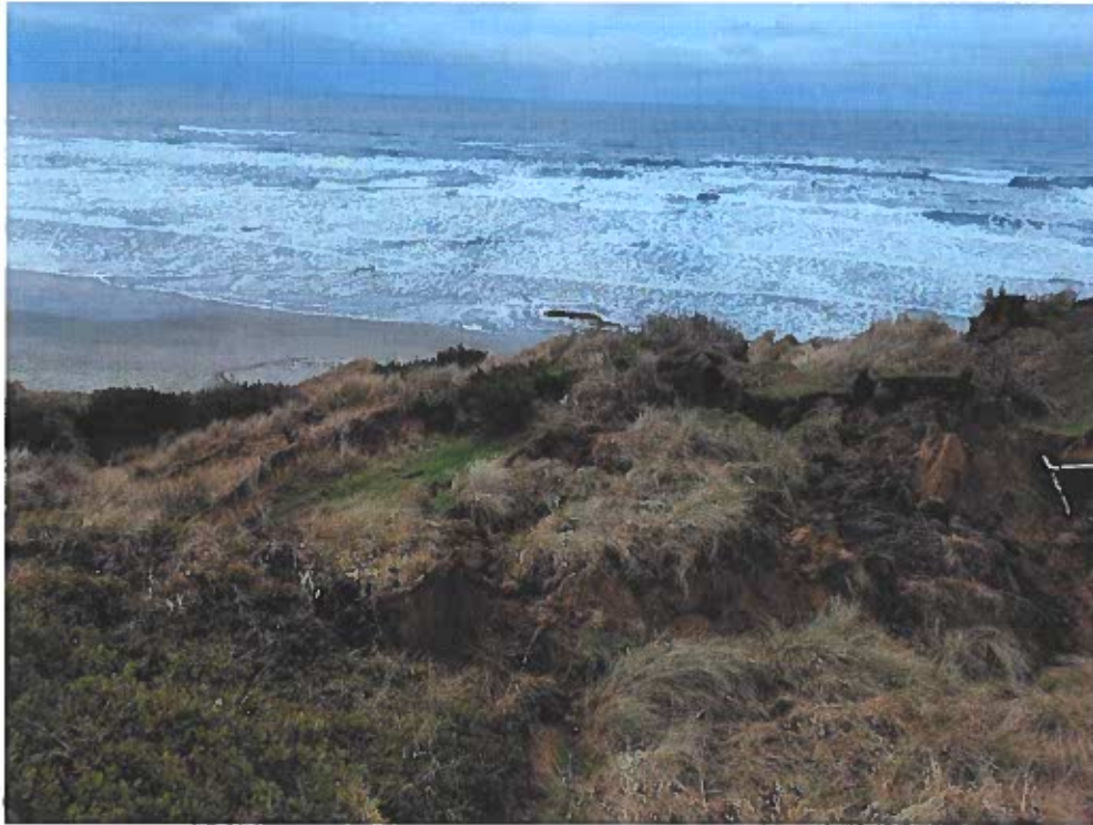
Photo 7. Failed slope at the top of the slide to the south of the building looking southwest.
