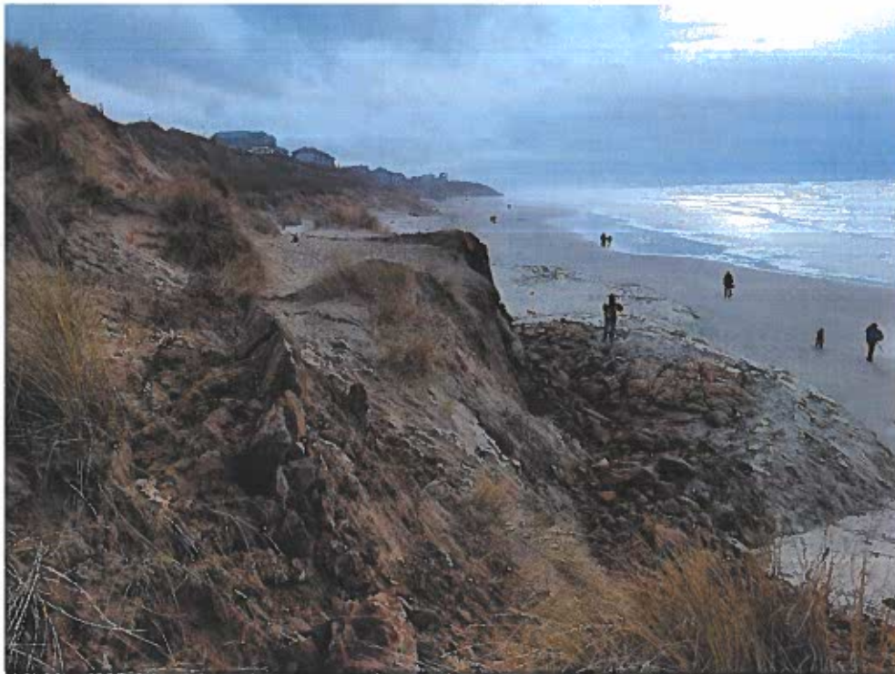
Photo 13. Heaved sand and debris at the toe in the southern portion of the slide looking south.
