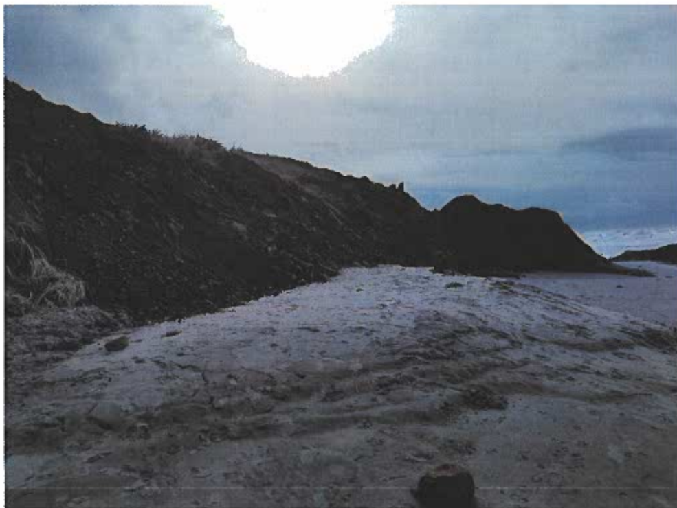
Photo 10. Debris and heaved sand at the toe in the northern portion of the slide looking south.
