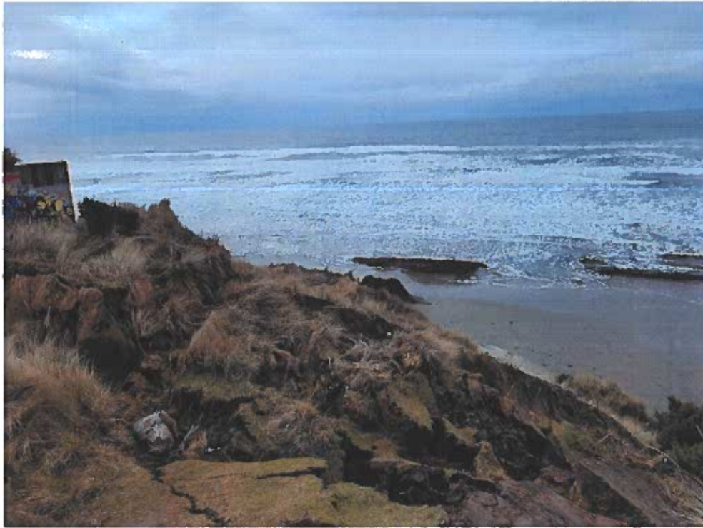
Photo 5. Failed slope at the top of the slide to the north of the building looking southwest.
