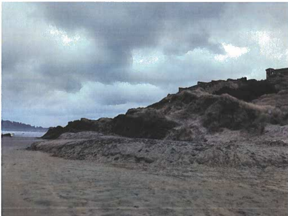
Photo 14. Heaved sand at the toe in the southern portion of the slide looking north.
