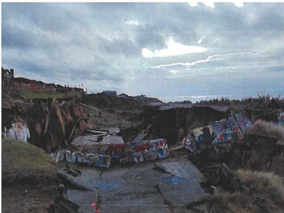
Photo 2. Head scarp and former building area looking south.
