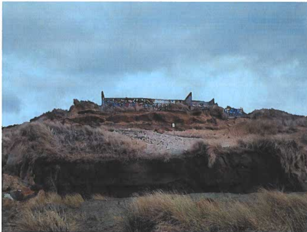
Photo 8. Sand and bedrock exposed on the slide surface below the building looking east.
