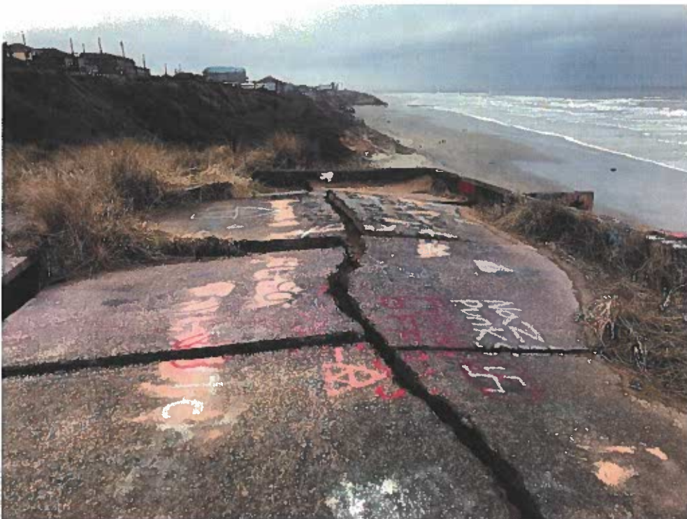
Photo 4 Floor slab in the western portion of the building area looking south.
