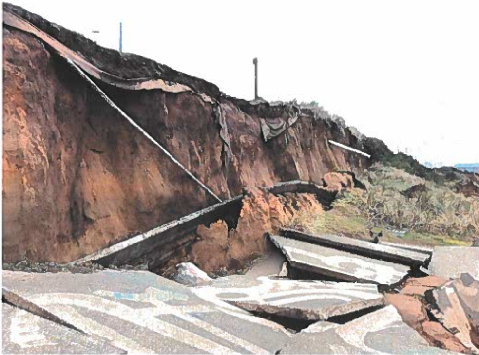
Photo 3. Soil exposed in the head scarp looking southeast.
