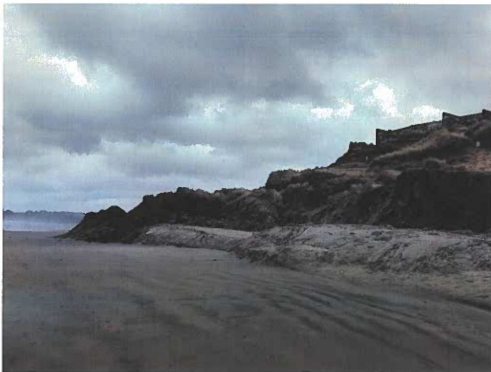
Photo 12. Heaved sand and debris at the toe in the central portion of the slide looking northeast.
