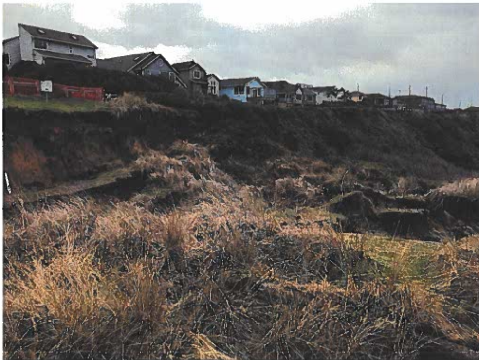
Photo 6. Failed slope and head scarp at the top of the slide to the south of the building looking southeast.
