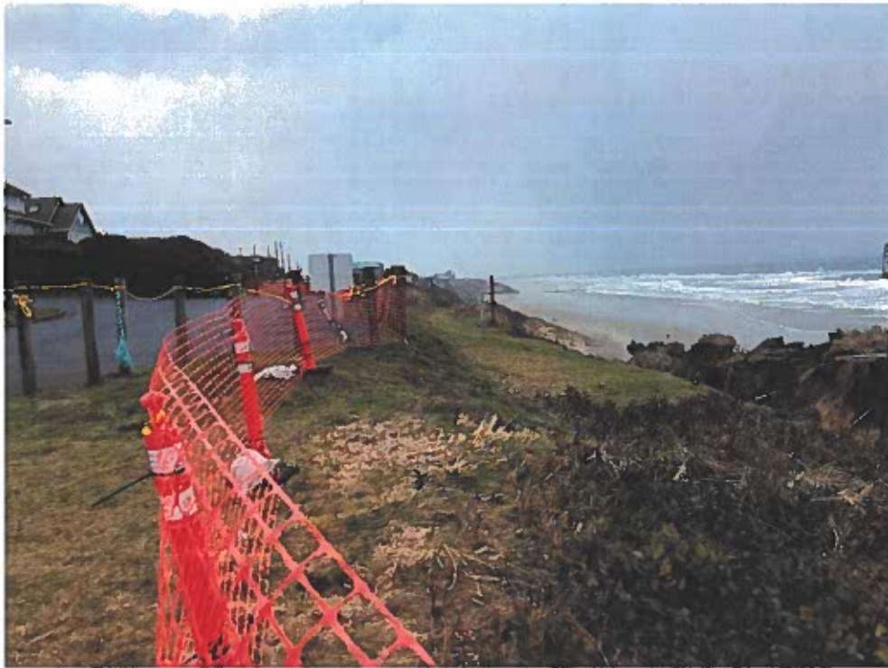
Photo 1. Proximity of the head scarp to the parking lot looking south.
