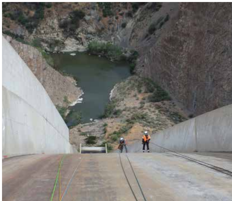
A rope-access inspection of a gated chute spillway.
