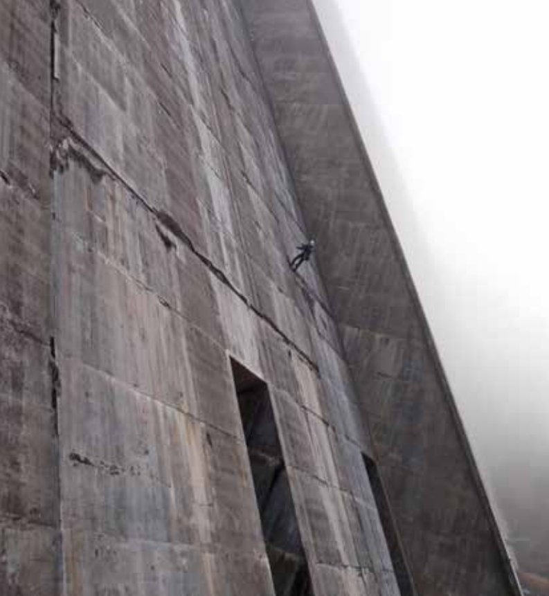
A rope-access inspection of a gated ogee spillway.
