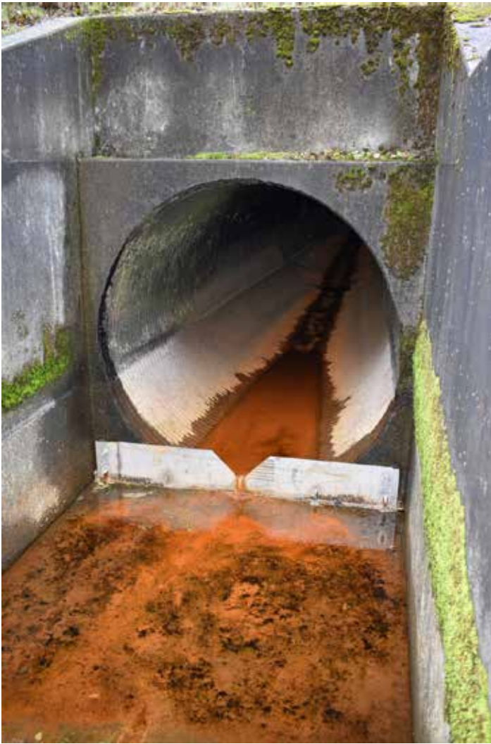
A dam outfall pipe showing evidence of seepage.
