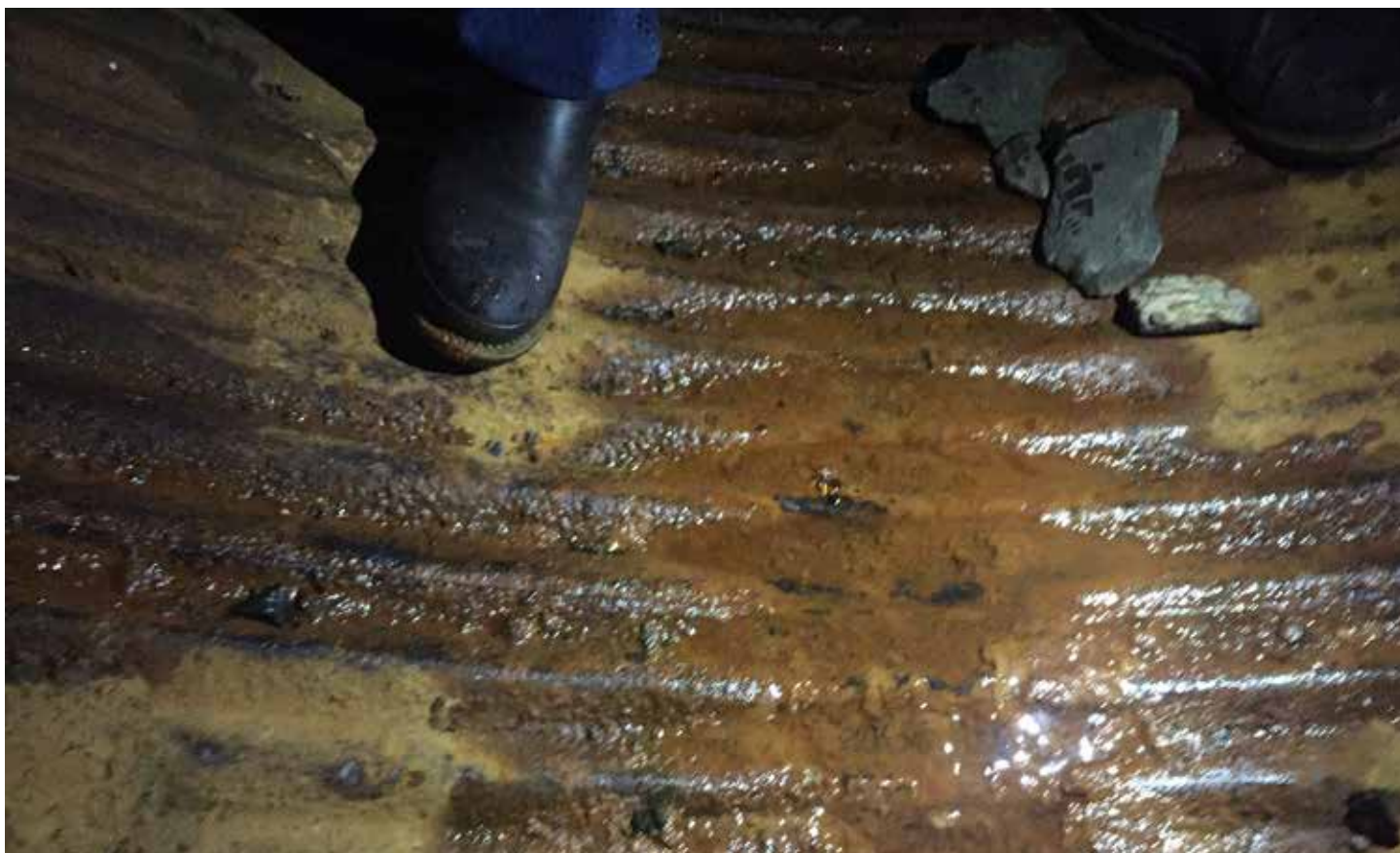
Corrosion and seepage on one of the dams' outfall pipes.
