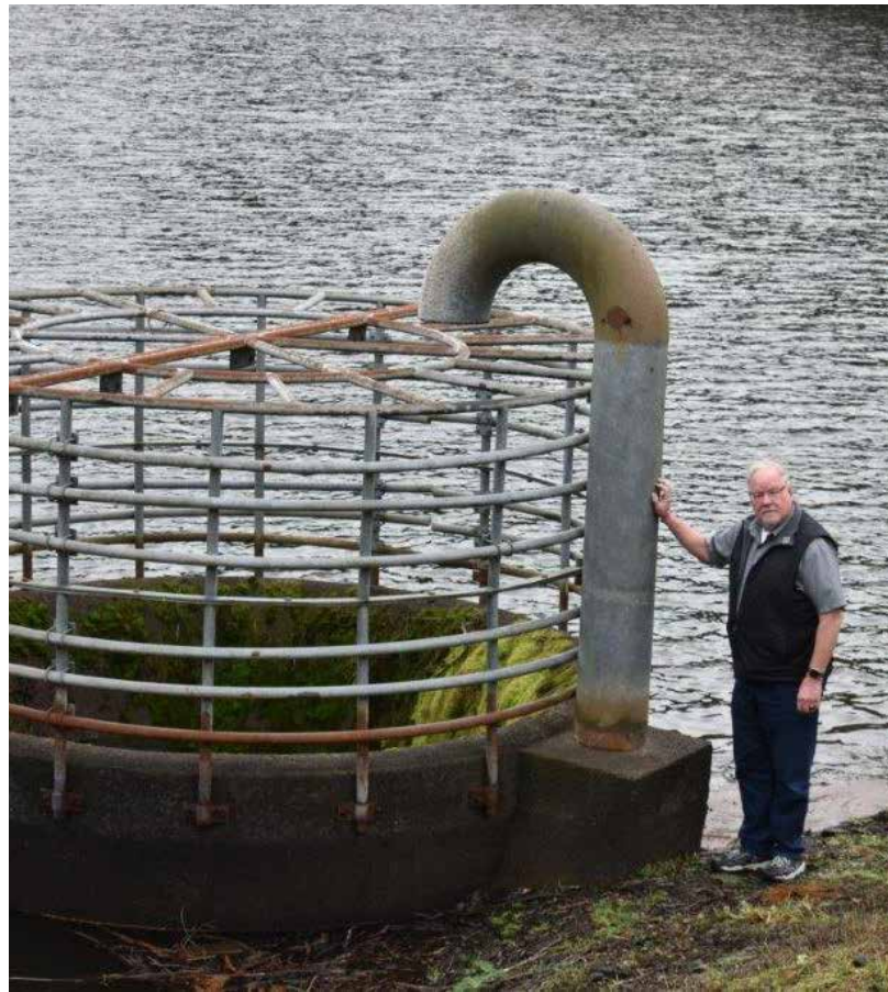
A bellmouth spillway at one of Newport's dams.
