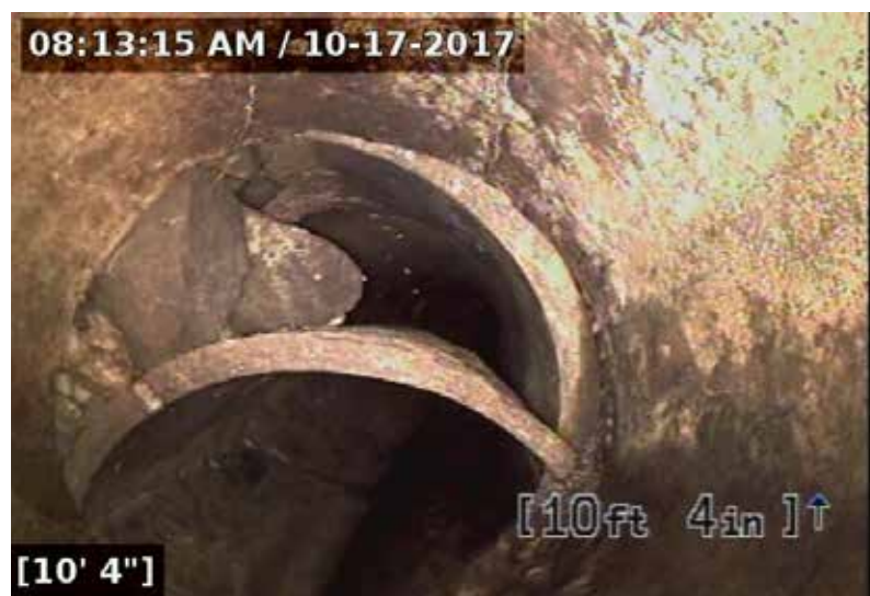
An underdrain inspection reveals a broken and displaced clay underdrain.
