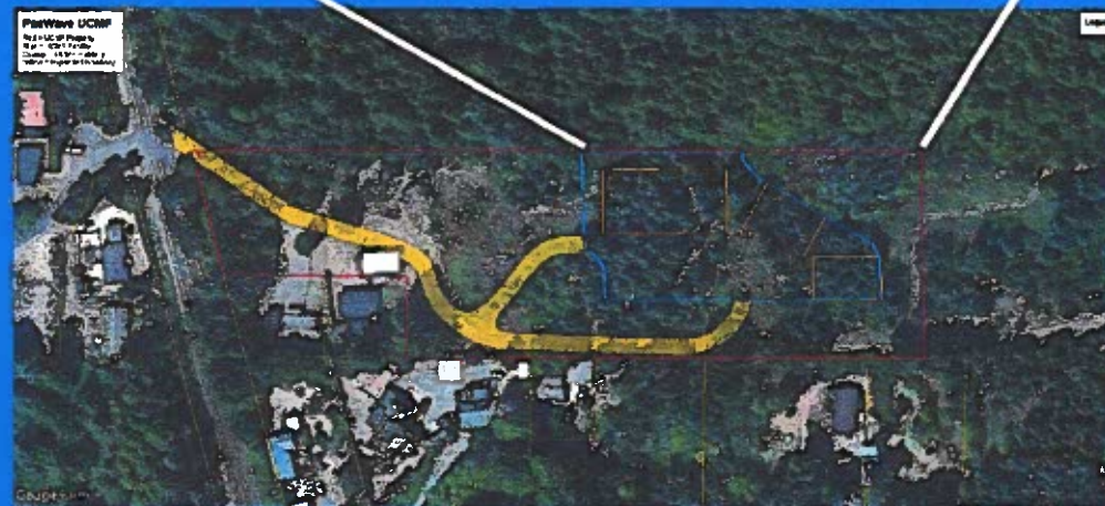
Utility Connection and Monitoring Facility “UCMF”
