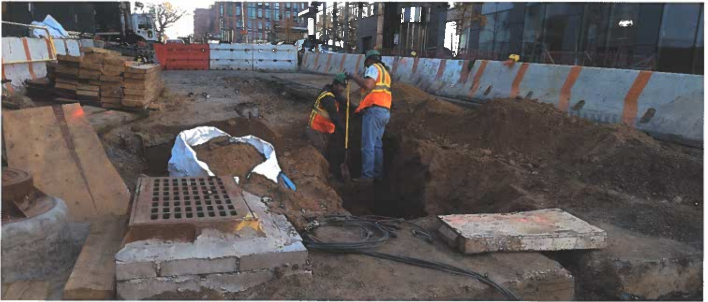
Excavations for a water main replacement.
