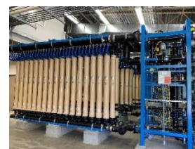
New Water Treatment Plant Filtration Rack
