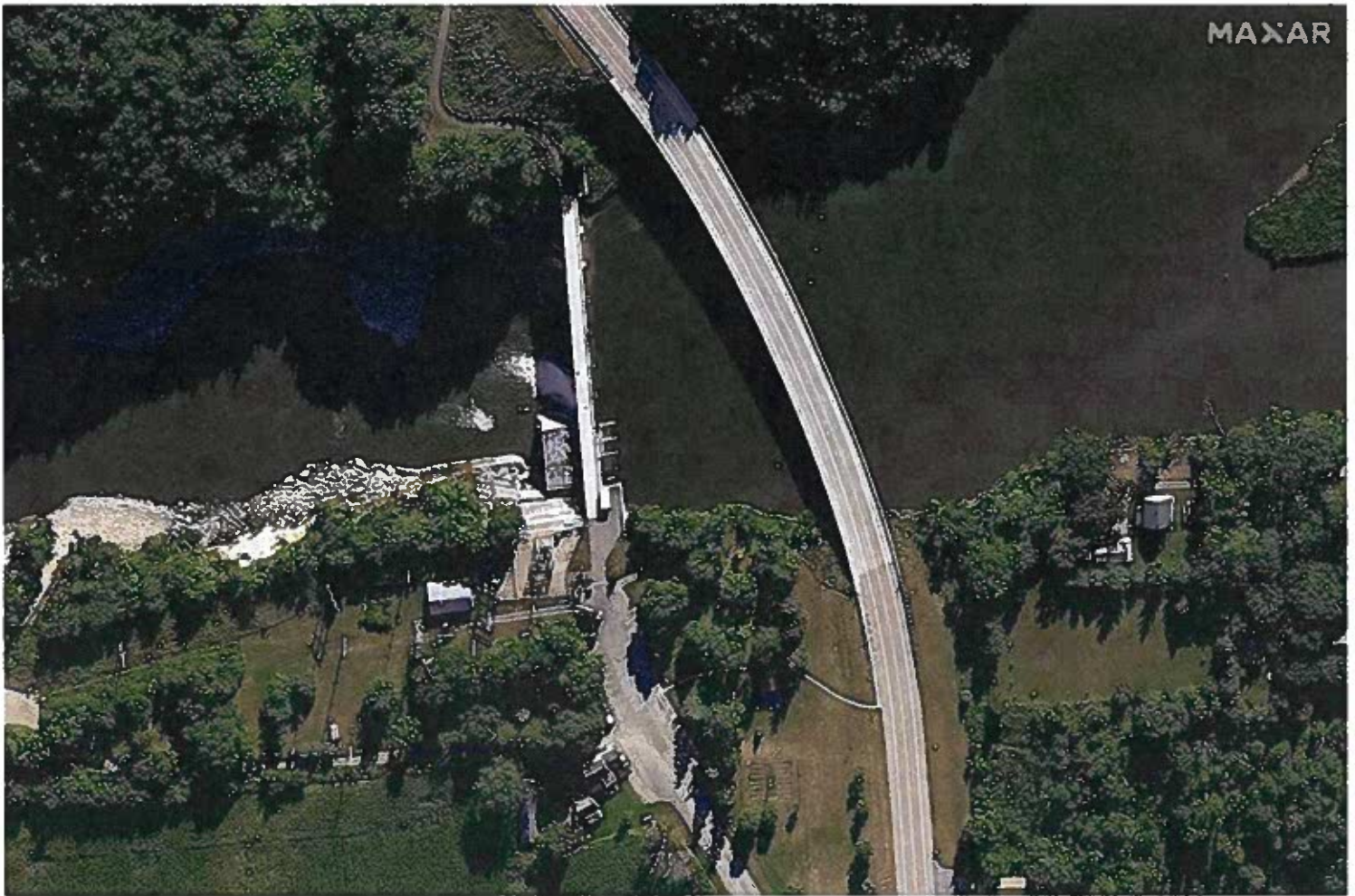
— Views of the Rapidan Dam on Sept. 6, 2011, and on June 26, after floodwaters overcame parts of the structure. Maxar Technologies via AP
