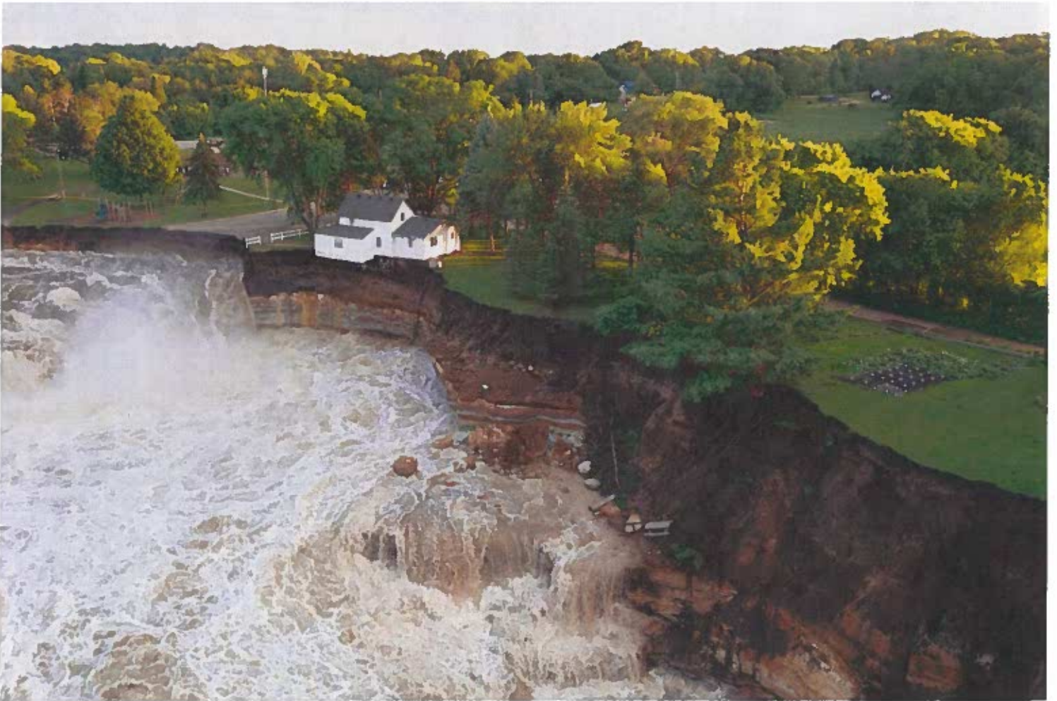
— A riverside home seen on Tuesday before it partially collapsed, near at the Rapidan Dam in Minnesota. Andrew Weinzierl / AW Aerial via AP
