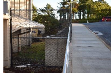
SE Benton and 10th Street Sidewalk and Retaining Wall
