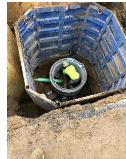
NW Grove Street Sewer Project
