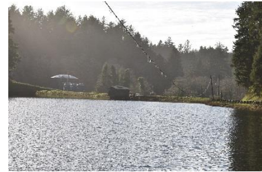
Big Creek Lower Dam
