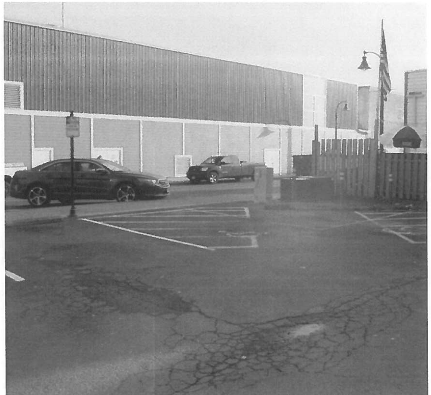
Fatigue Cracking – Abbey Street Lot (2016)
