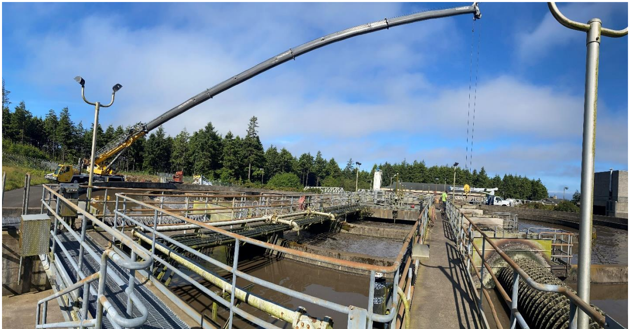
Wastewater Treatment Plant Motor Removal
