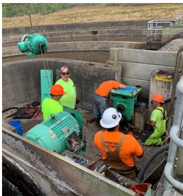
WWTP Crew Replacing the Aeration Basin Equipment
