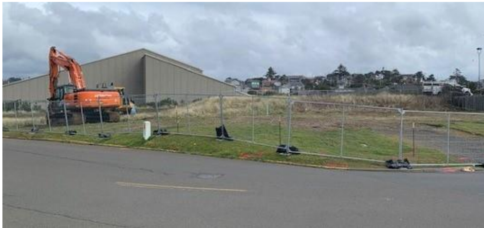
Breaking Ground for The Whaler Inn Expansion
