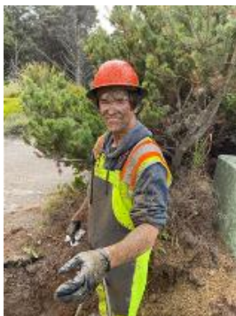
WWC crew using the Jetter
