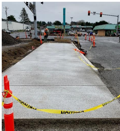
Harbor Freight Sidewalk Construction Project
