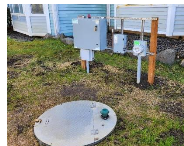
Wastewater Collection Meter Installation
