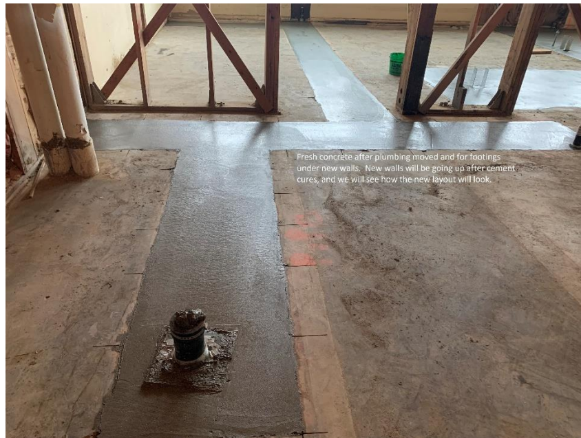
Performing Arts Center Renovation
