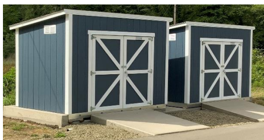
Big Creek Trash Enclosures
