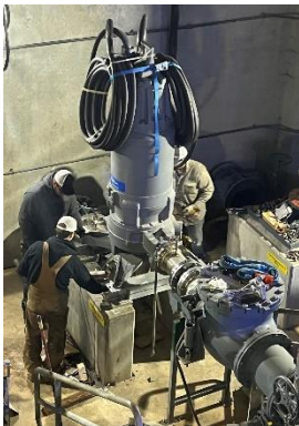
North Side Pump Station Installation
