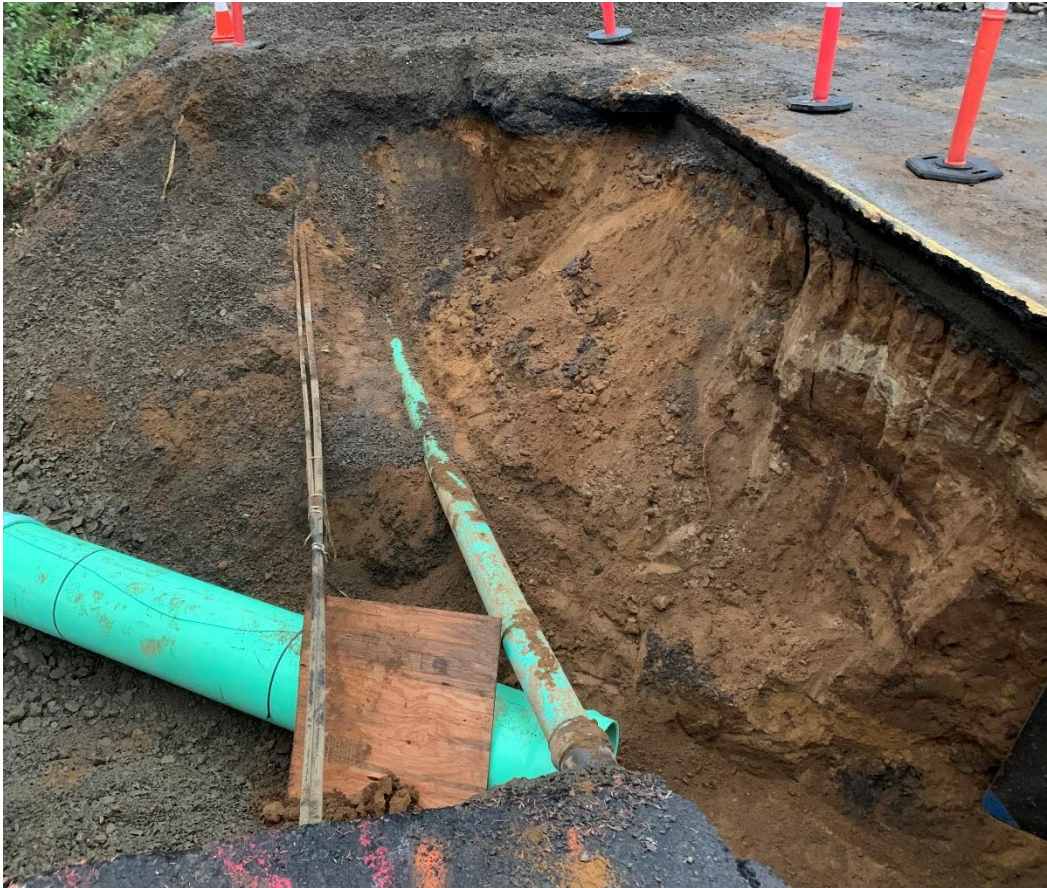
Oceanview Drive Sanitary Sewer and Storm Pipe Replacement
