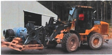
New Pump Installation at the Main Influent Wastewater Pump Station
