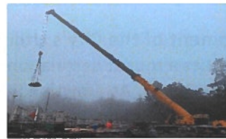
Wastewater Treatment Plant Clarifier Installation
