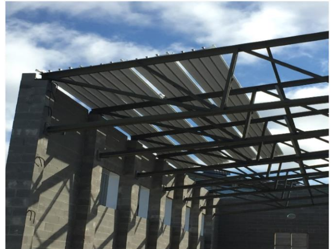
Aquatic Center roof trusses and decking installation.
