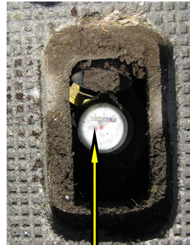
Most meters are now electronic meters; yours may look a bit different but all have a "face" reader display. Open the cover to reveal the meter display.
