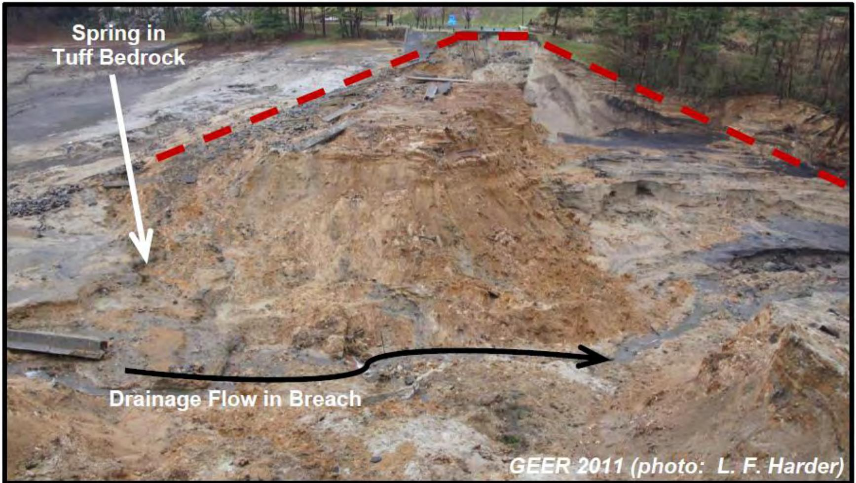
Figure 8: View of Breach in Fujinuma Main Dam from Right Abutment
