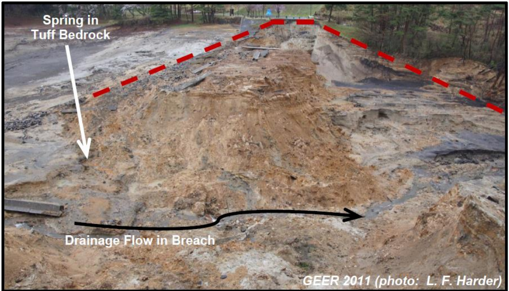
Figure 8: View of Breach in Fujinuma Main Dam from Right Abutment (N37.3014°, E140.1957°, April 23, 2011)
