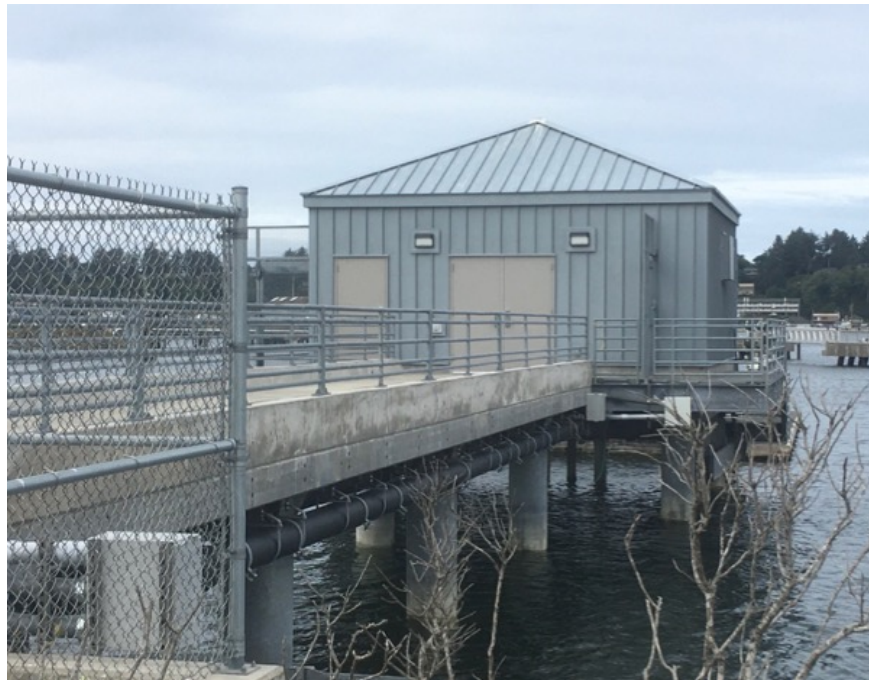
HMSC Intake Facility
