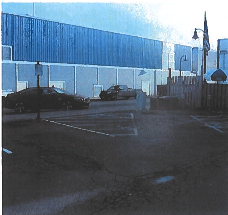
Fatigue Cracking – Abbey Street Lot (2016)
