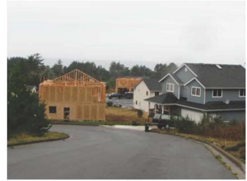
N.E. 71st and Avery Housing Construction
