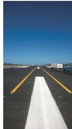
Airport Runway Reconstruction
