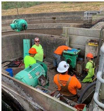
WWTP Crew Replacing the Aeration Basin Equipment
