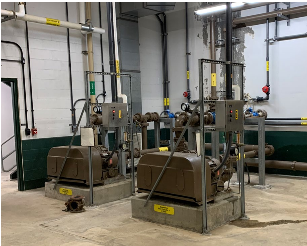
Figure 3-4. Centrifuge feed pumps
