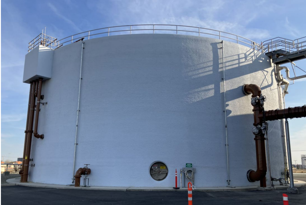
Figure 7-3. Anaerobic digester
