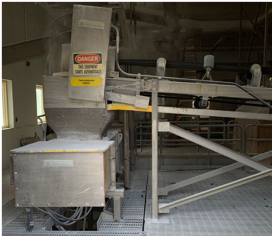
Figure 3-6. RDP lime stabilization equipment
