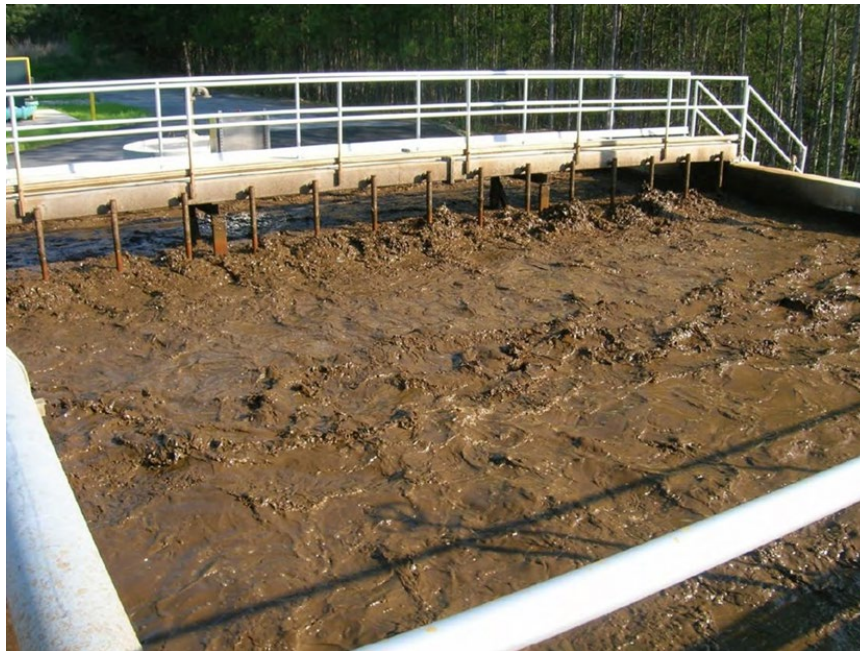
Figure 7-2. Aerobic Digester
